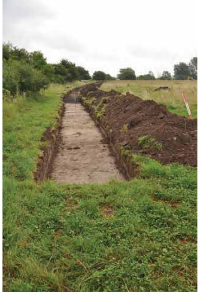
Searching for drainage pipes, the sticks mark the pipes.
