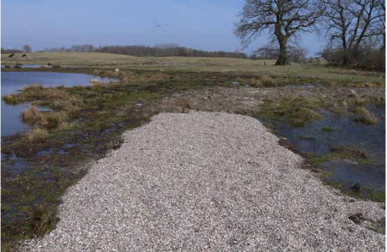
Fish barrier consisting of a 50 cm layer of gravel. This layer of gravel prevents fish migration between ponds, but permits percolation of water.
