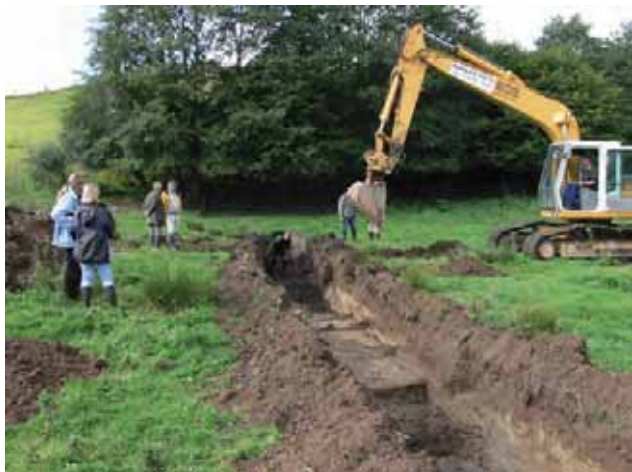
A test hole is dug in order to examine the pedological conditions and to choose the right placement of a pond.
