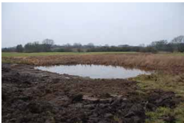
An old pond is cleaned and enlarged at one side.
