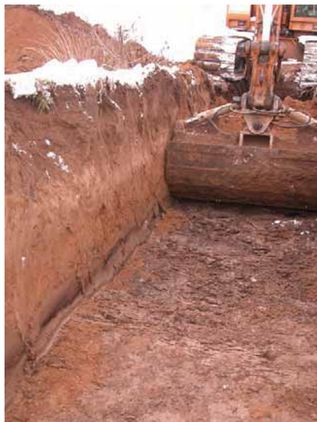
The soil conditions at this site (pure clay) are good for a pond feeding only on precipitation.
