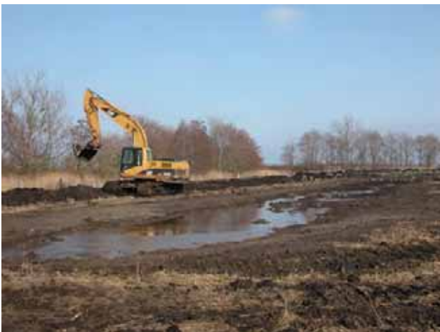
A dam is build to create a shallow flooding.
