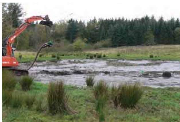
Before the mud is removed the pond is pumped dry by an excavator hydraulic pump (12cm 3 /min).
