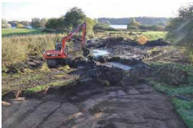
Organic material and mud is a source of nutrients and should thus be removed from a pond.
